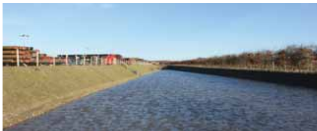
Surface water runoff pond at Fordoun, Aberdeen.
